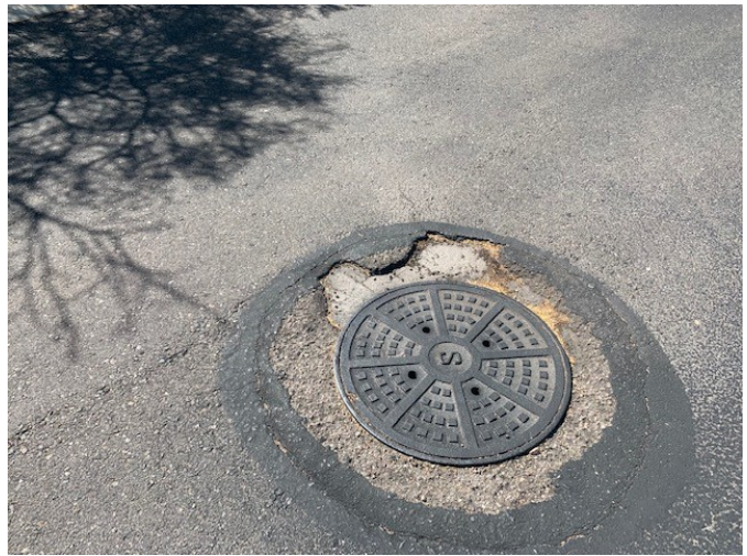
Asphalt cracks
